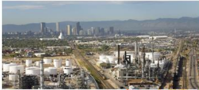
Suncor Refinery Area
